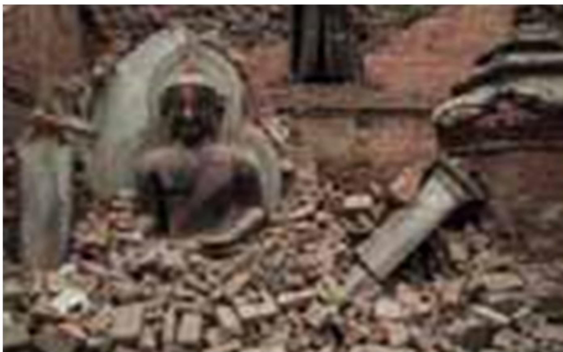
■ Figure 2.23 Temple damaged during the earthquake
