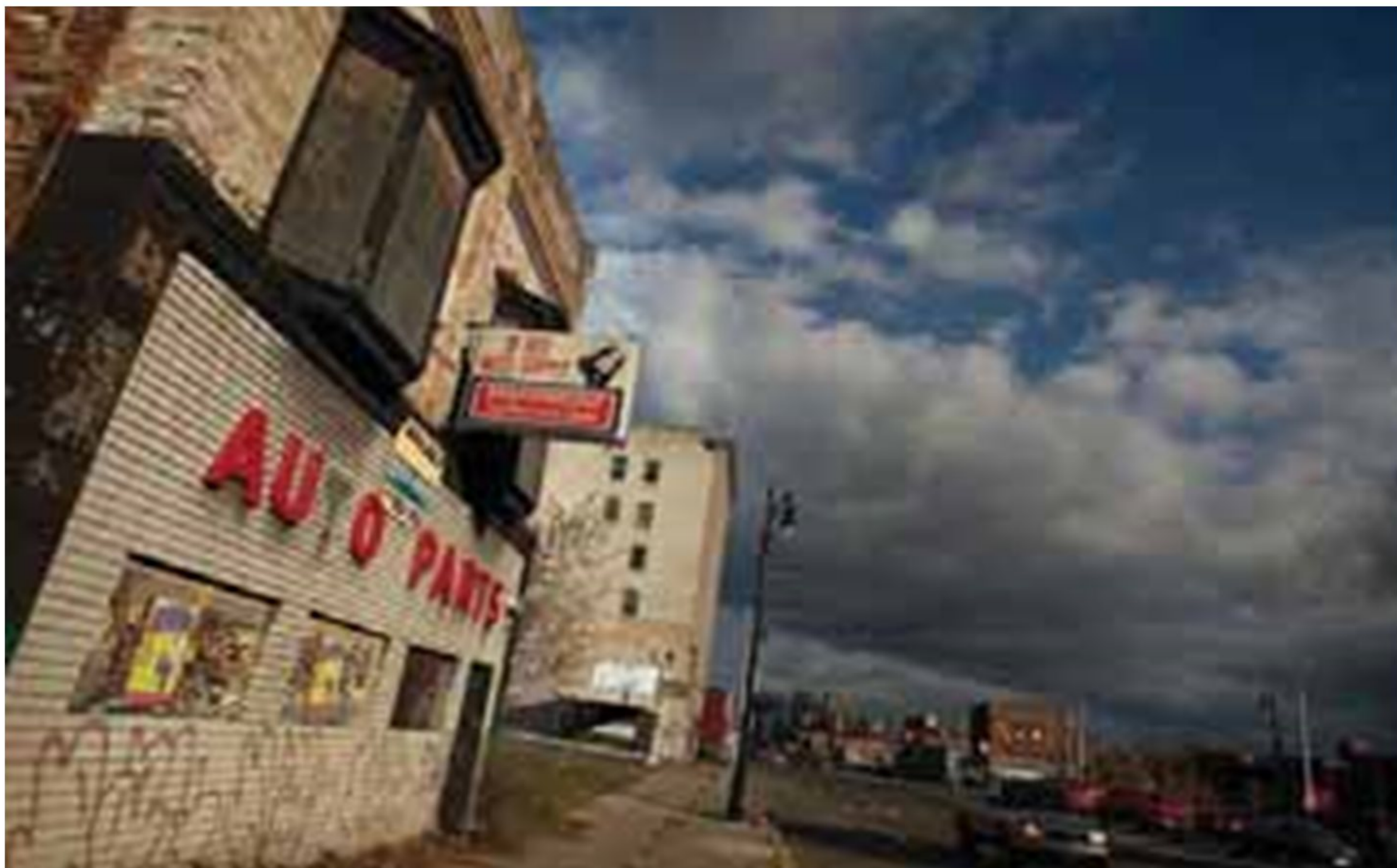
■ Figure 4.21 Abandoned buildings in downtown Detroit, 2008
