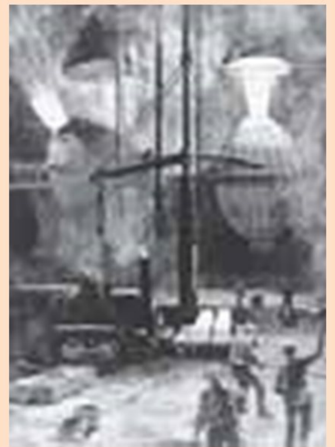
■ Figure 6.8 A steel mill from the era of the Industrial Revolution in the UK
