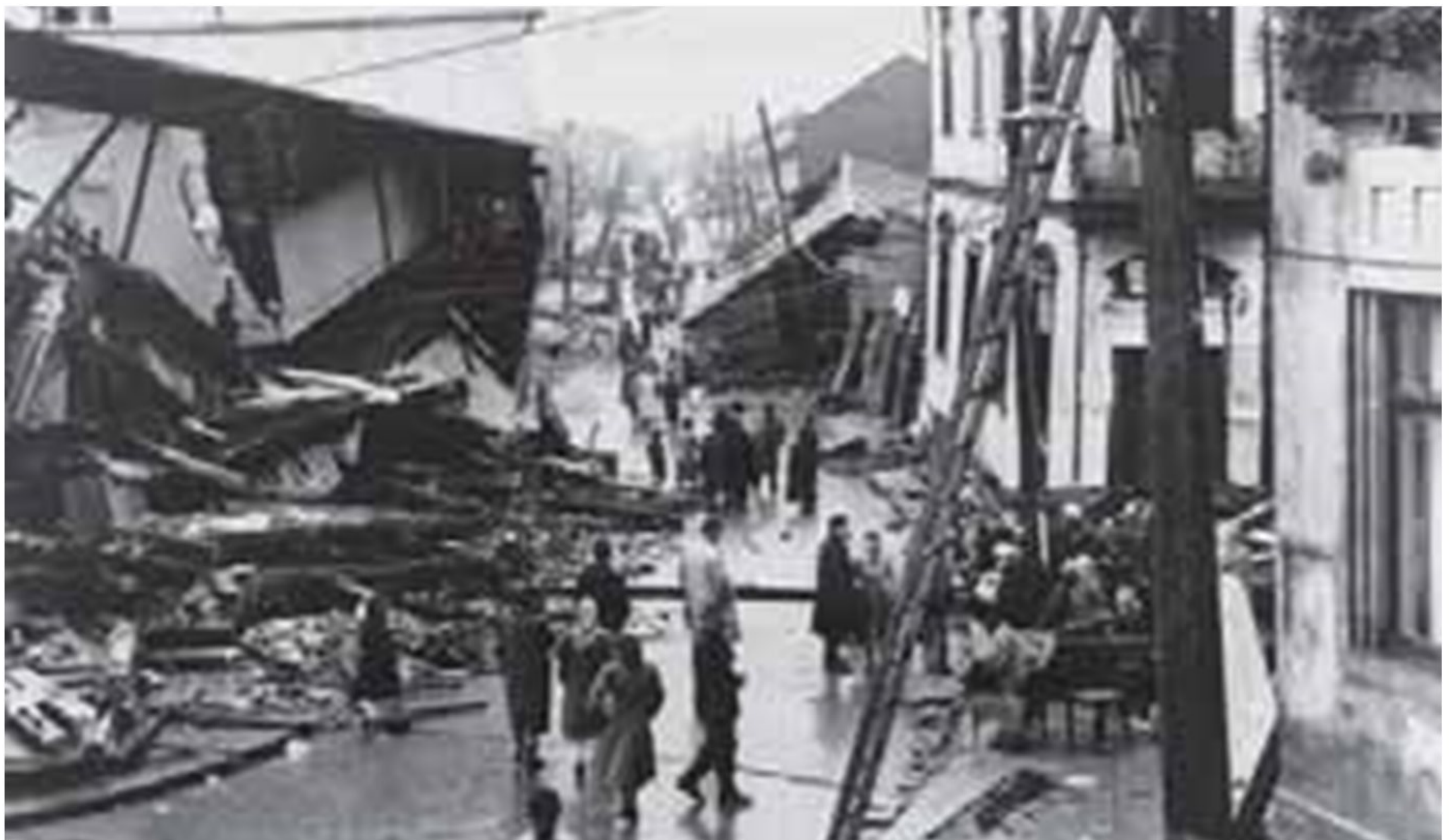
■ Figure 2.14 Damage done during the Valdivia Earthquake in Chile, 1960
