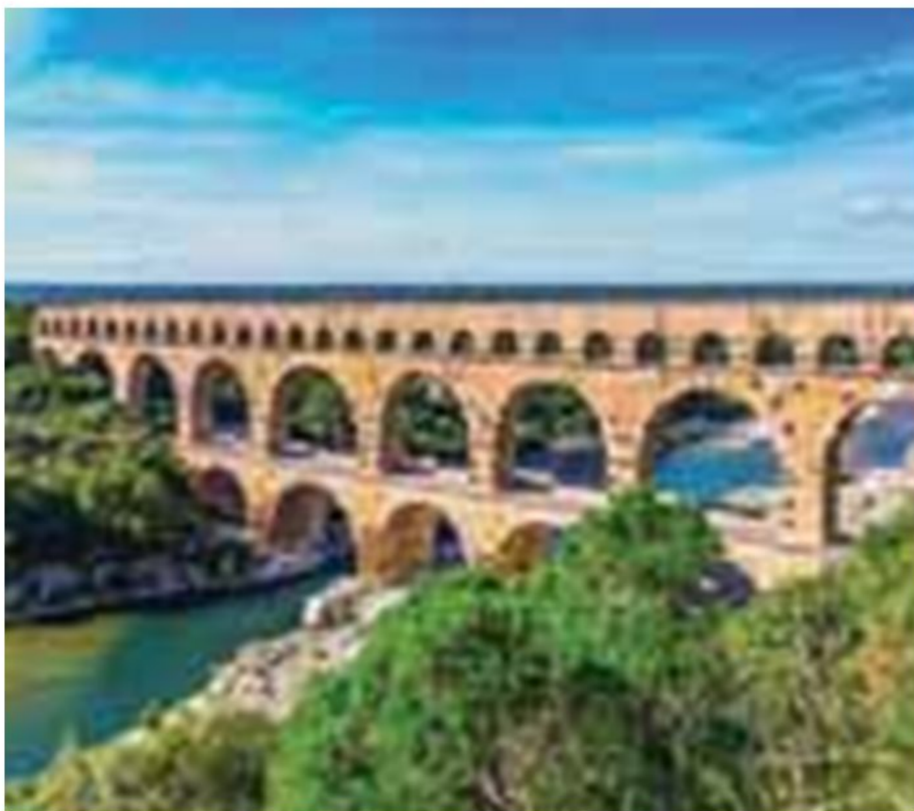
■ Figure 3.7 Roman aqueduct built in France, c. 19BCE
